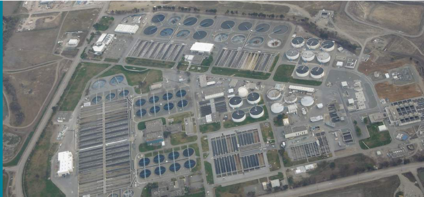
Figure 25.1 Sewage Treatment Plant (credit: "thekirbster"/flickr.com)
