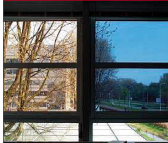
Electrochromic glazing going from coloured state (on the right) to bleached state (on the left).
