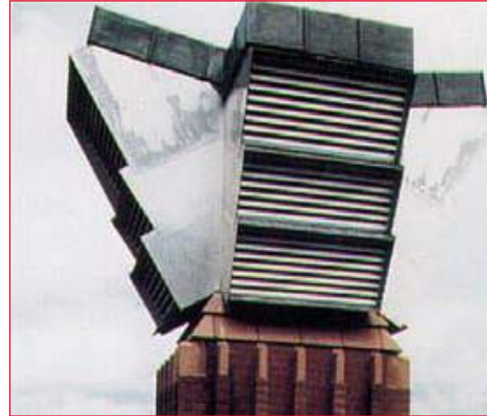
Ventilation stack, School of Engineering, Leicester (arch. Short Ford & Associates).
