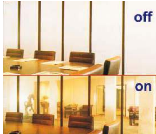
Smart windows: a liquid crystal film is sandwiched between the panes. 1
