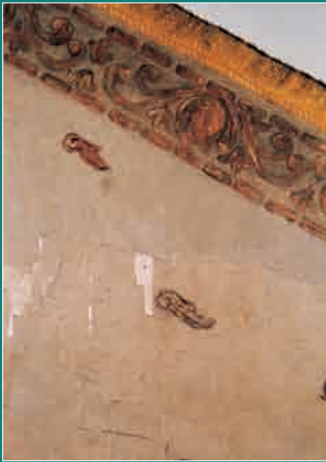
FIGURE 12 Detail of the lower swallow-tail with the reconstruction of the missing decoration (upper part) and the conserved original decoration (lower part)
