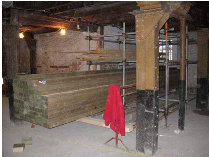
Figure 5 A designated timber storage area
