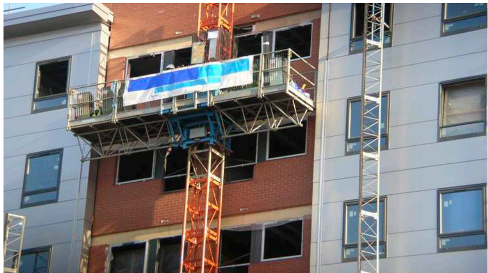
Figure 14 A mast climbing work platform
