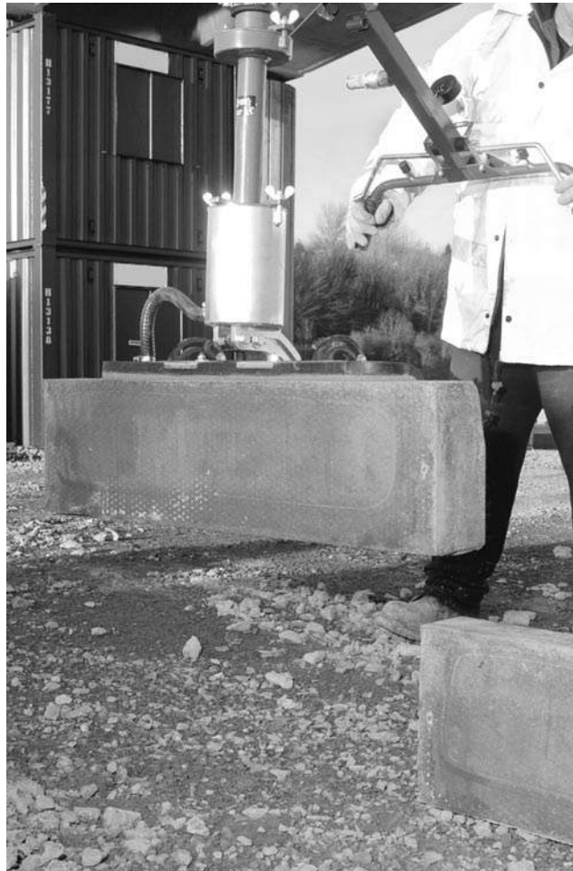
Figure 38 Handling kerbs using a vacuum lifter
