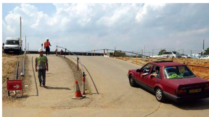
Figure 34 Pedestrians are segregated from vehicles on this slope
