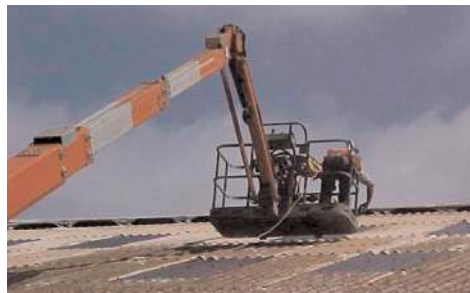
Figure 26 A mobile elevating work platform being used to replace a roof sheet
