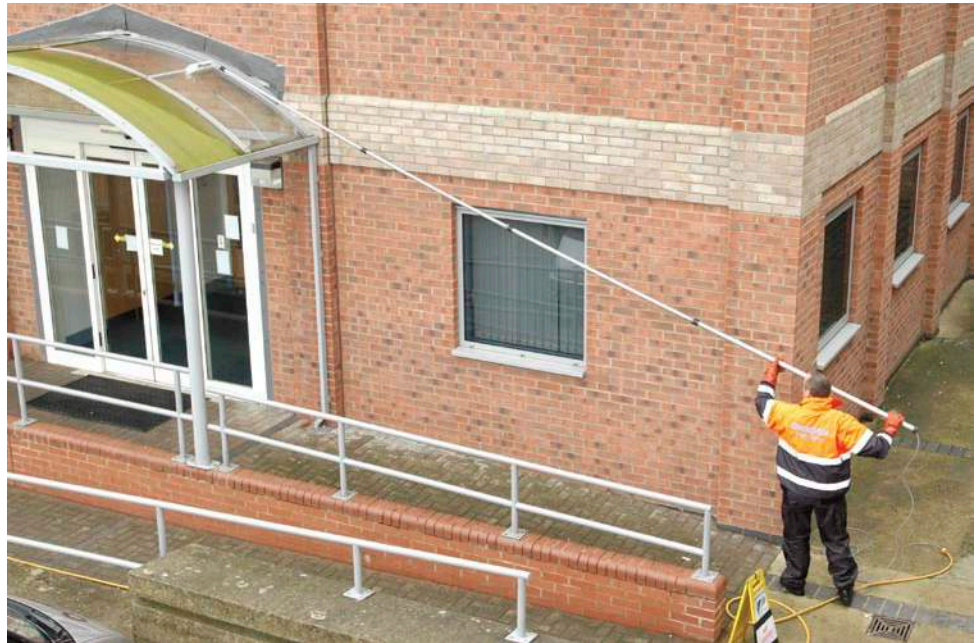
Figure 8 Using a long pole to avoid working at height
