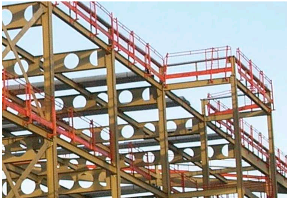
Figure 28 Edge protection installed with the steelwork
