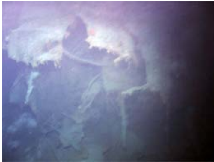
Figure 158: The break in the Fore-castle Deck looking down towards the ship's keel [251]
