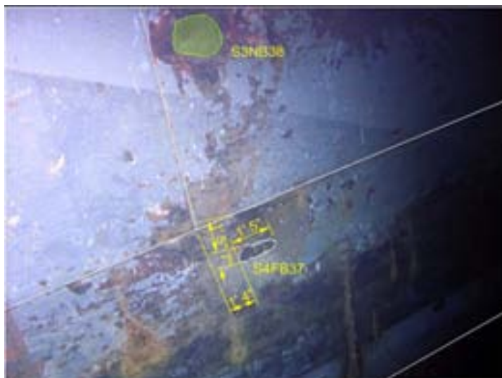
Figure 342: In vicinity of No. 1 Cable Passage, Platform deck [309]
