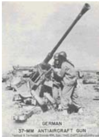
Figure 86: 3.7cm AA gun (Flak 18 and 36) [151]
