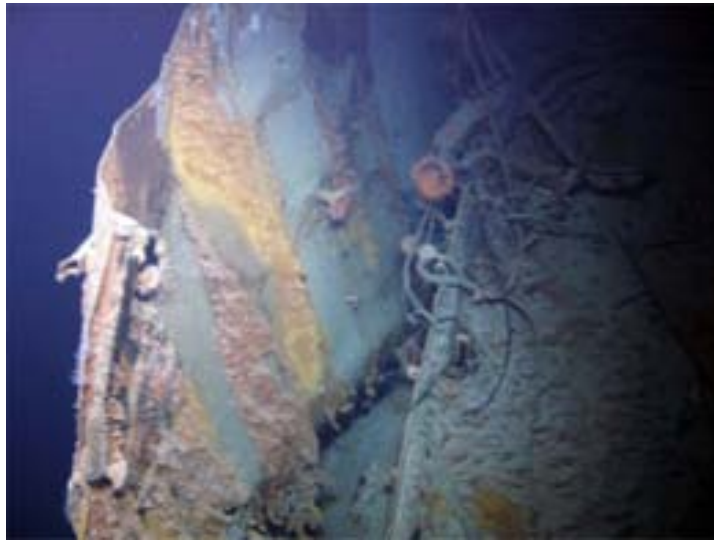
Figure 122: Starboard side of main hull bent upwards [178]
