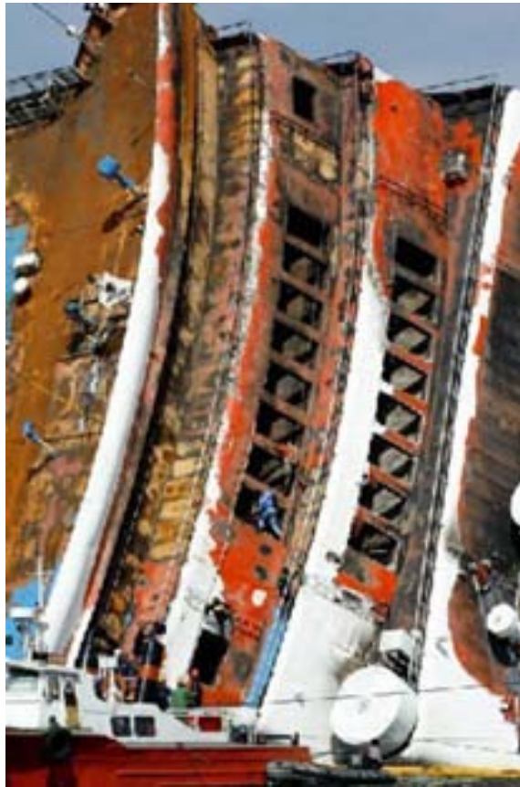
Figure 19: Fire damage to Superferry 14 [38]
