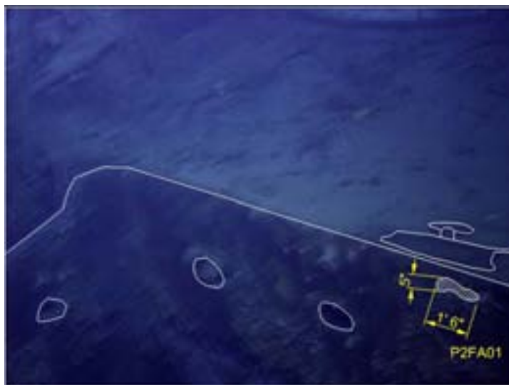
Figure 286: In vicinity of CPO's Mess, Upper deck on port side [339]
