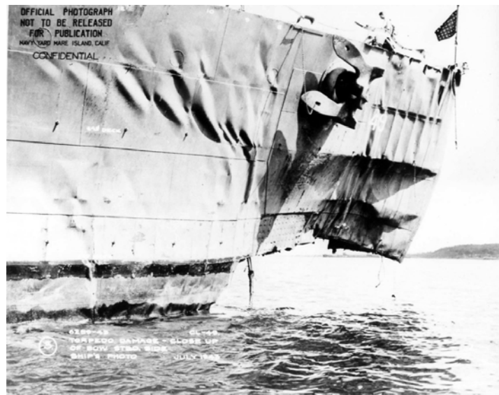
Figure 118: Torpedo damage to USS St. Louis in July 1943. This damage has penetrated through the hull [174].
