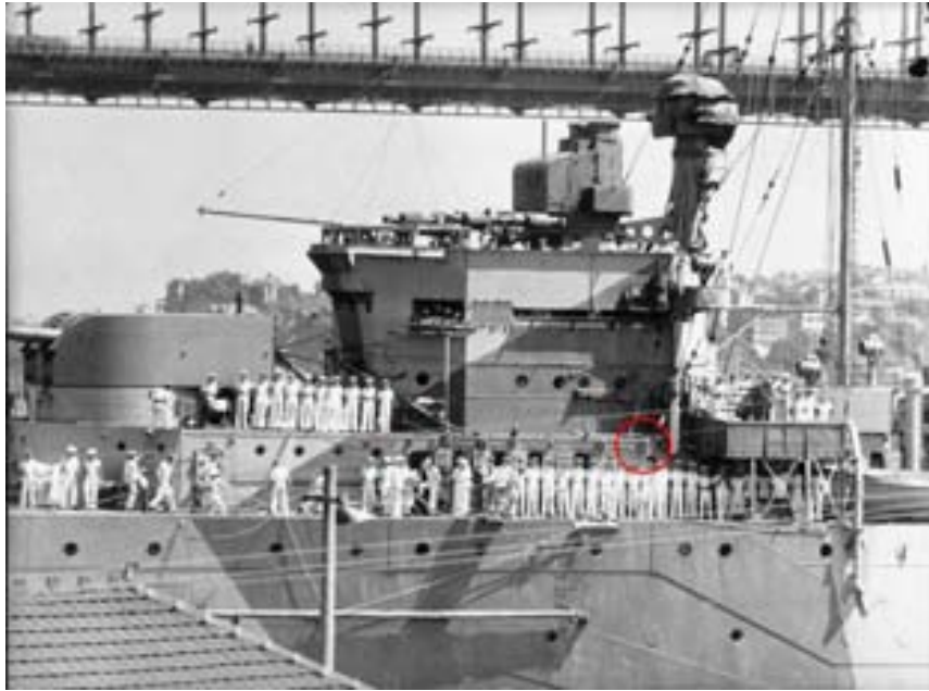
Figure 54: Location of a typical ventilation inlet on the Fore-castle deck, port side [97]
