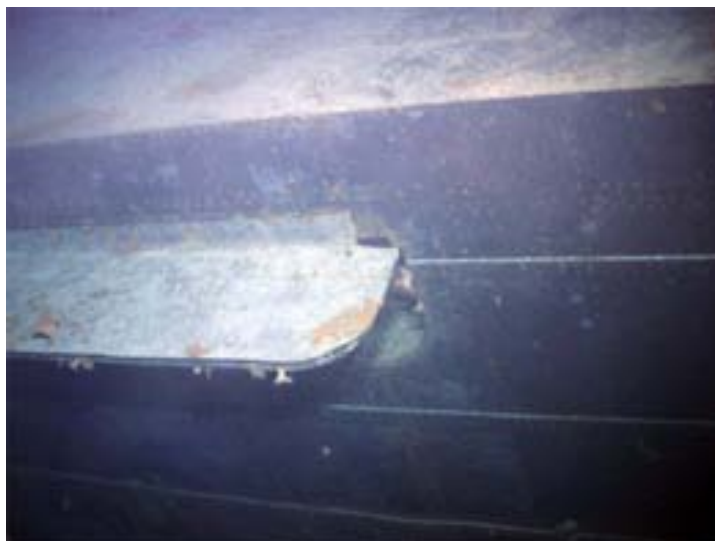
Figure 104: Above water torpedo flap port side [165]
