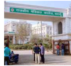
Work has been stalled at the Government Medical College, Badaun, for over a year as the matter is before a tribunal. ADITYAGUPTA/X
