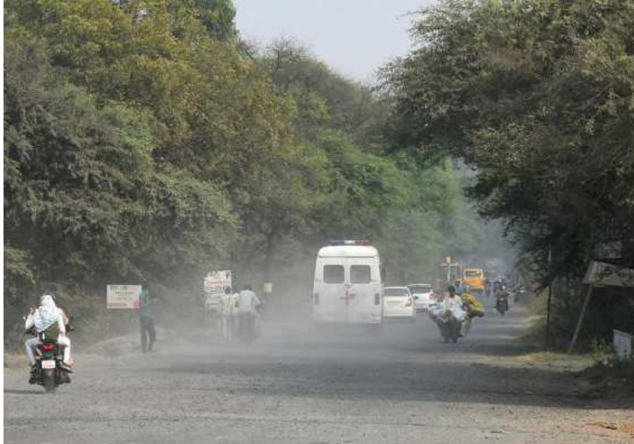
Pressing issue: A dusty and damaged road leading to the Bhojeshwar temple. A.M.FARUQUI
