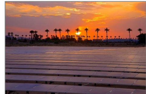
4.56mW Ironwood Solar project
