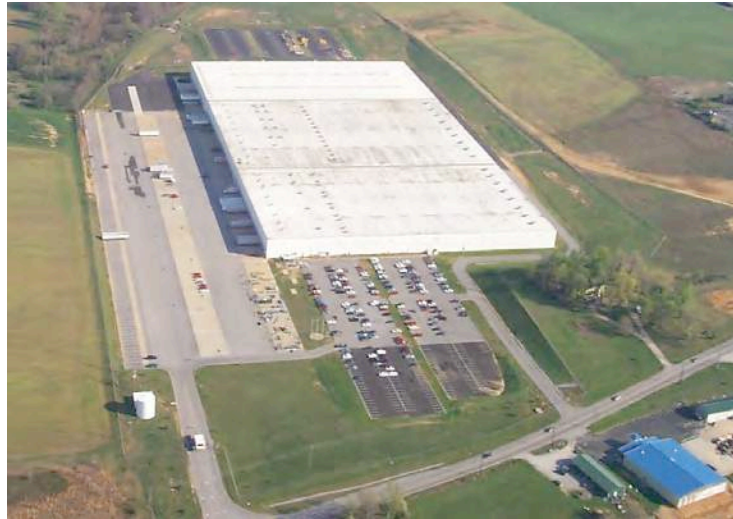
Figure 17.1: This Amazon.com distribution center is typical of the large, high-volume DCs in North America.
