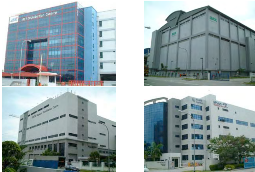
Figure 17.4: Multi-story warehouses are common in Singapore, Hong Kong, and Japan where land is expensive.
