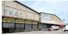
Figure 17.7: To shed rain, this roof is steeply angled, which makes it more difficult to utilize vertical space within.
