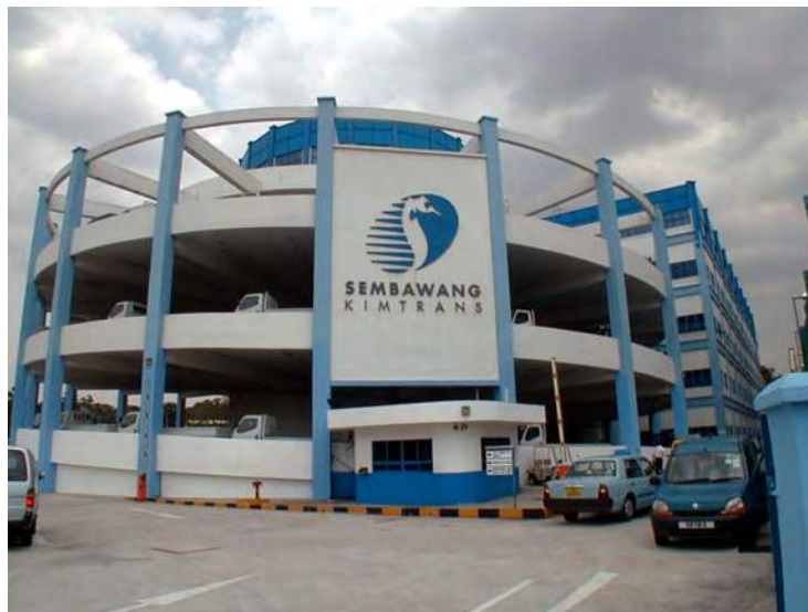
Figure 17.5: Multi-story warehouse with no automation but accessibility provided by a spiral truck ramp.
