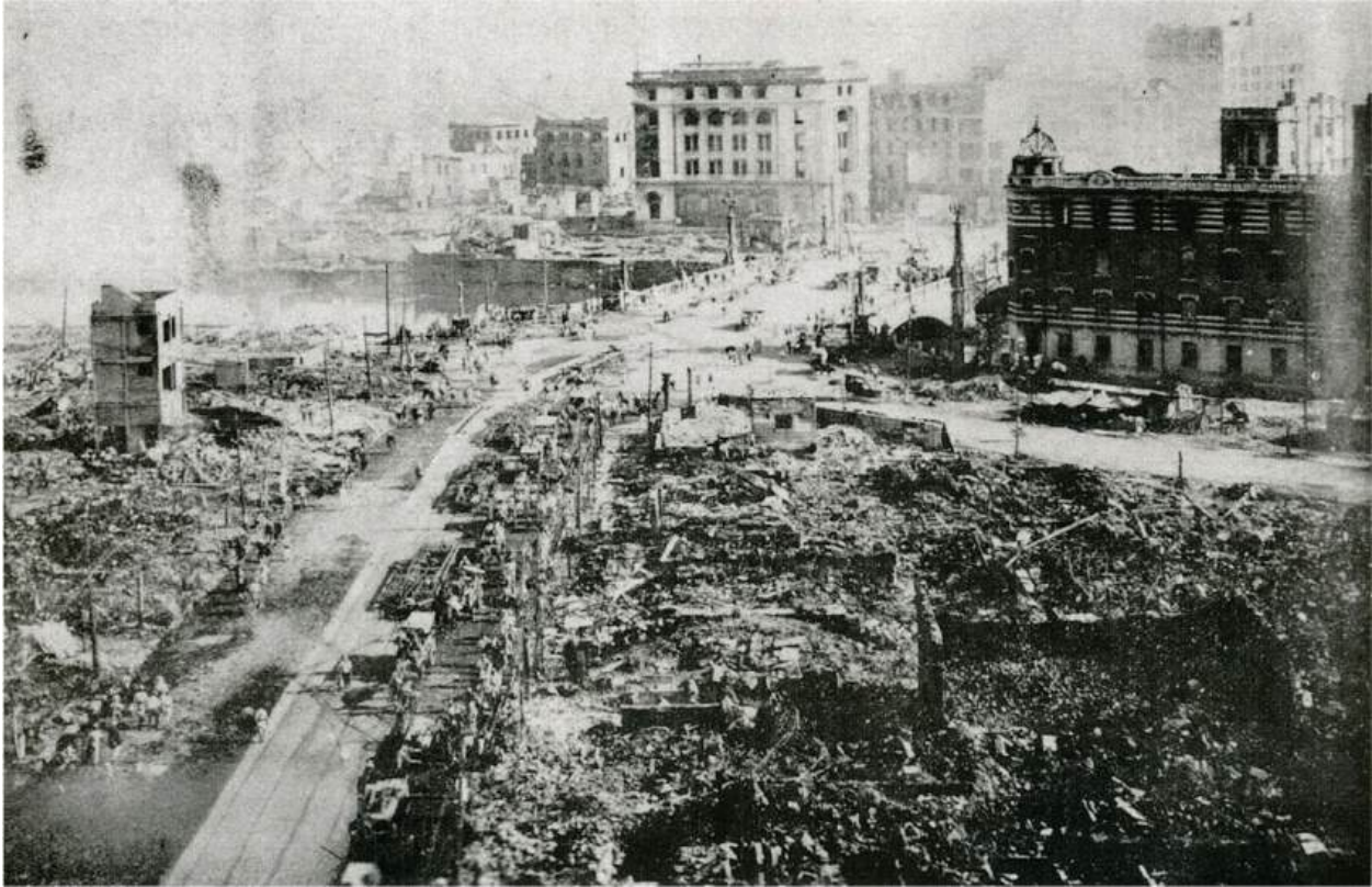
FIGURE 12.18 A City Destroyed. This 1923 photograph shows the extent of destruction in Tokyo caused by the Great Kanto Earthquake in 1923. (credit: modification of work “The Great Kanto Earthquake” by “urbz”/Flickr, CC BY 2.0)
