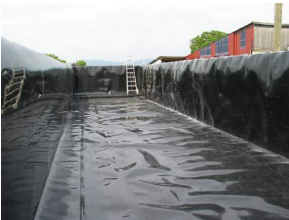
(c) ASSESS-GPR after installation of the pond liner
