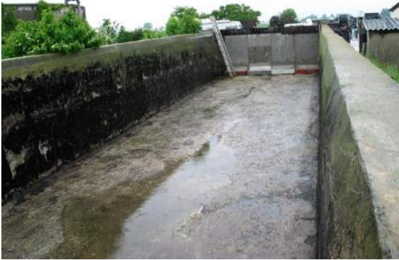
(a) ASSESS-GPR site before construction. View towards start of GPR profiles
