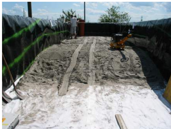
(d) ASSESS-GPR during construction
