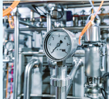
Pneumatic and hydraulic installations
