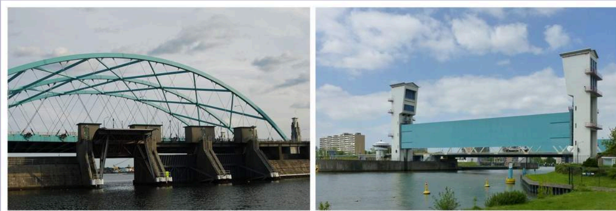
Figure 8.4.6 The Fox Point Hurricane Barrier in Providence, RI, USA (left) and the surge barrier on the Hollandse IJssel river in southern Holland. (Fox Point by Marabela (Marc N. Belanger) (Own work) [Public domain], via Wikimedia Commons; Dutch barrier by Mark Voorendt (Own work) [CC BY-SA 4.0], via Wikimedia Commons).
