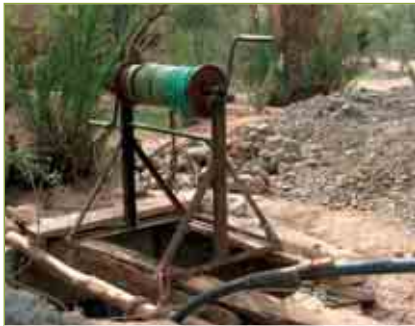
Building a well, Morocco
