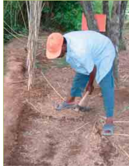
Step 1: Digging the pit
