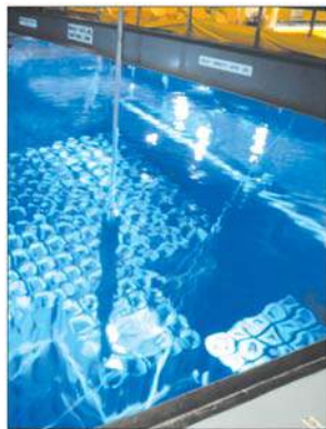
Typical spent nuclear fuel storage pool.
