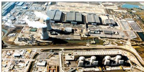
Uranium enrichment plant at Tricastin, France. This enrichment plant alone is large enough to more than meet the needs of all nuclear reactors in France.
