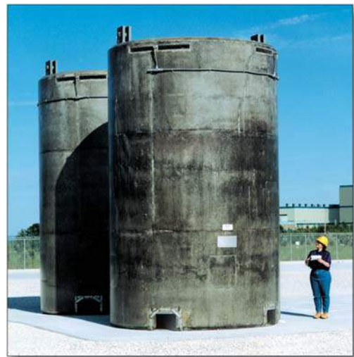
Dry storage of spent fuel.
