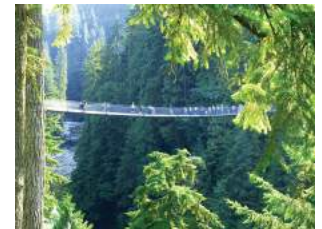
Figure 10.5 Capilano River Bridge
