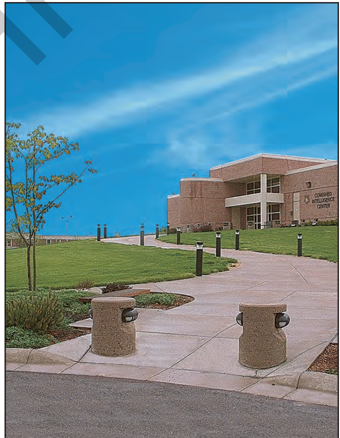
This entrance sidewalk is also the handicap access ramp. Light bollards restrict vehicular movement, as well as allow pedestrian access.
