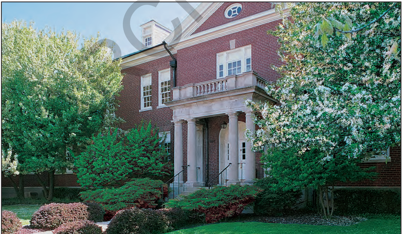
Shrubs and ornamental flowering trees frame the entrance and enhance the character of this historic building.
