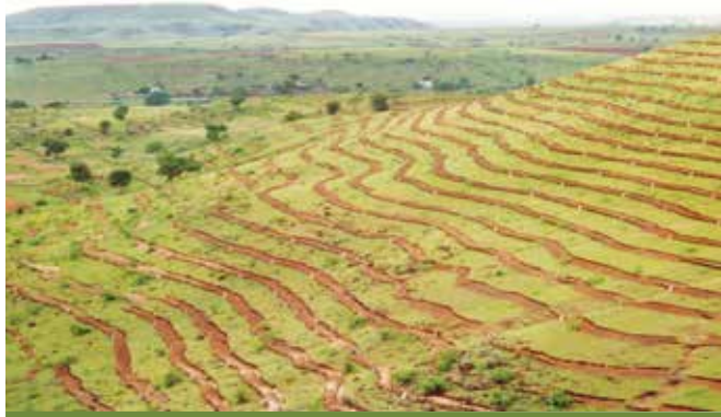
Contour trenching for runoff collection
