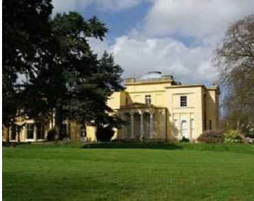
Figure 9 – Upton Hall, headquarters of the BHI
