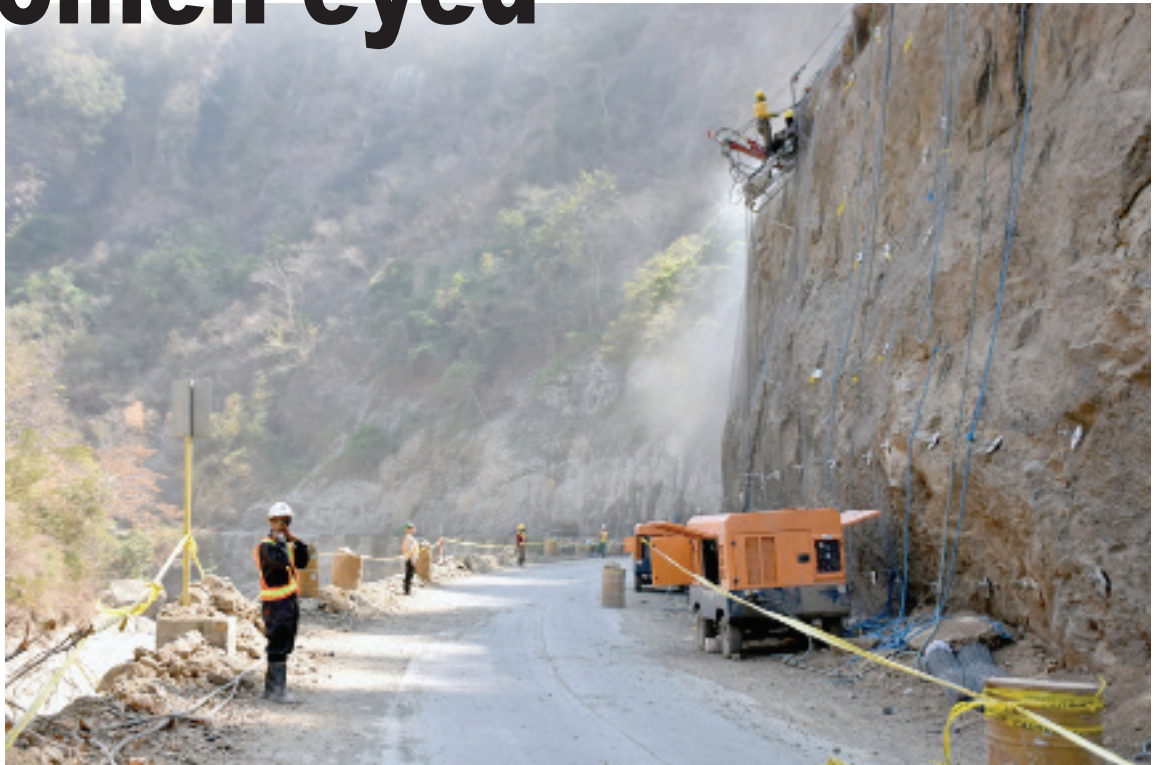
Kennon Rock net - Back to work. After the more than a week of opening the historic Kennon Road to the public, rehab works resume particularly at the rock netting of Camp 1 in Tuba, Benguet to ensure safety of the road once it opens to the public permanently./RMC PIA-CAR
