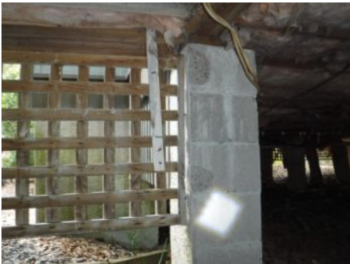
Pier (leaning)- Pier as pictured is leaning and structurally deficient. (at least three noted) Repair as needed.
