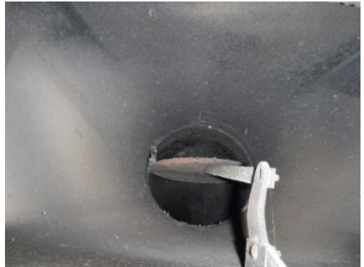
view up flue
