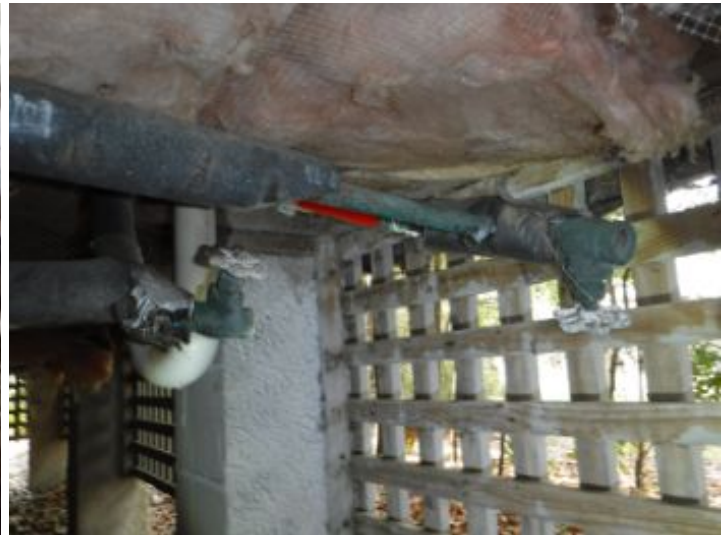
piping needs a little support here
