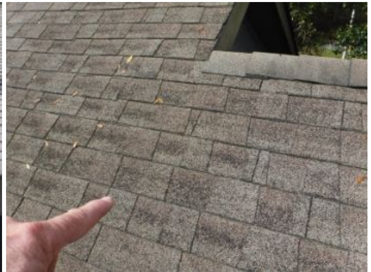
Nail pop pictured. Repair as needed to prevent moisture intrusion.
