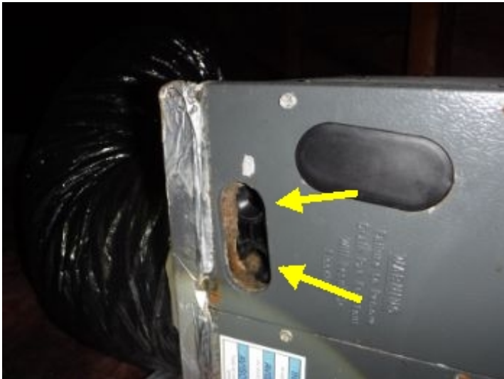
open ports allows air to escape; suggest adding plug
