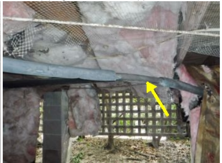
piping needs a little support here
