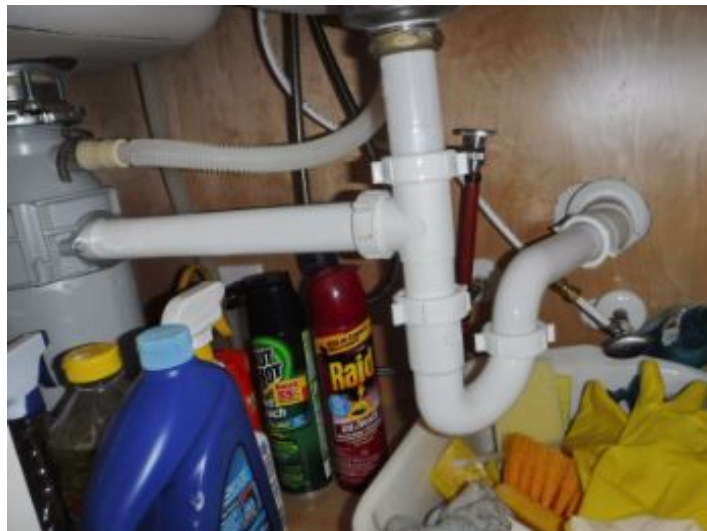
under sink view
