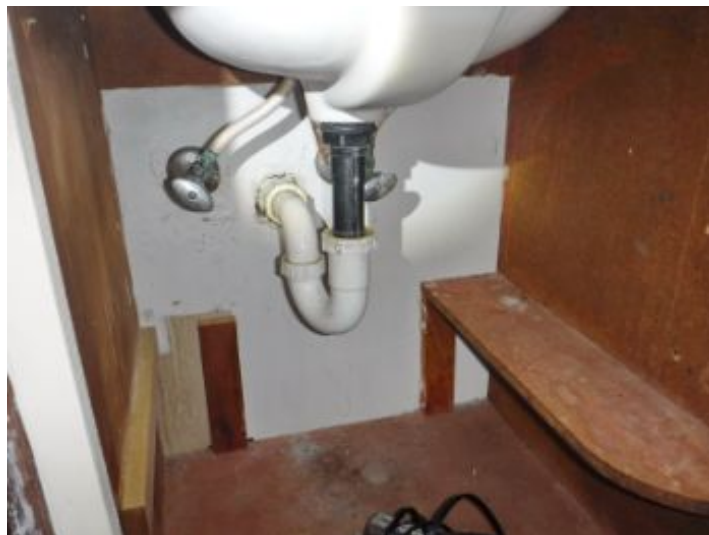
under sink view
