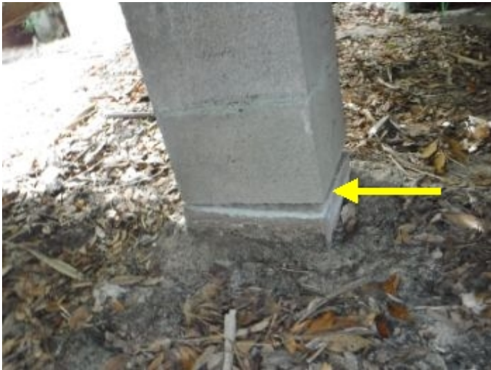
Pier (leaning)- Pier as pictured is leaning and structurally deficient. (at least three noted) Repair as needed.
