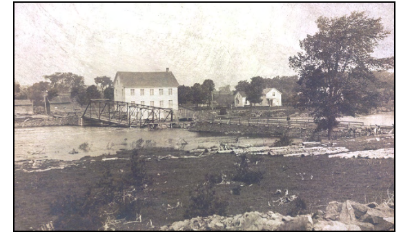
Mill at Andrewsville in 1904 and bridge failure. Parks Canada.
