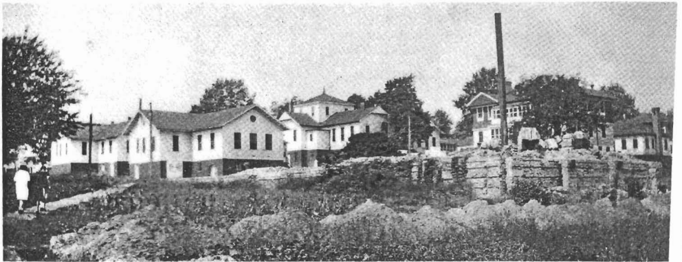
Frame Buildings—Erected between 1859-1898 for use as General Hospital Units
