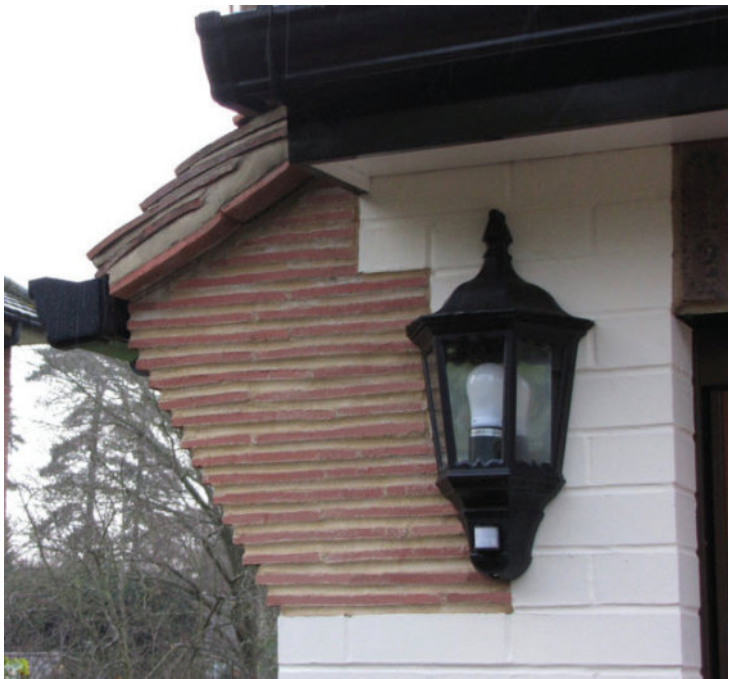
Where a gable intercepts with an eave
