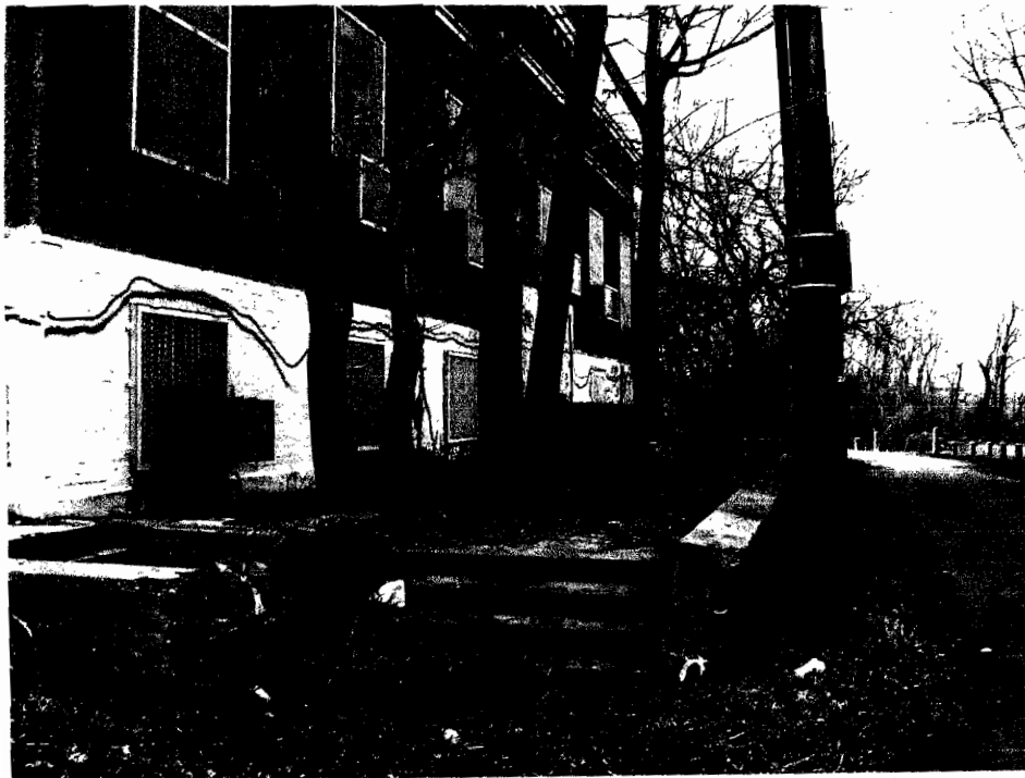
Stone steps at south end of walkway along east façade of school – lead to front steps to former main entrance.
