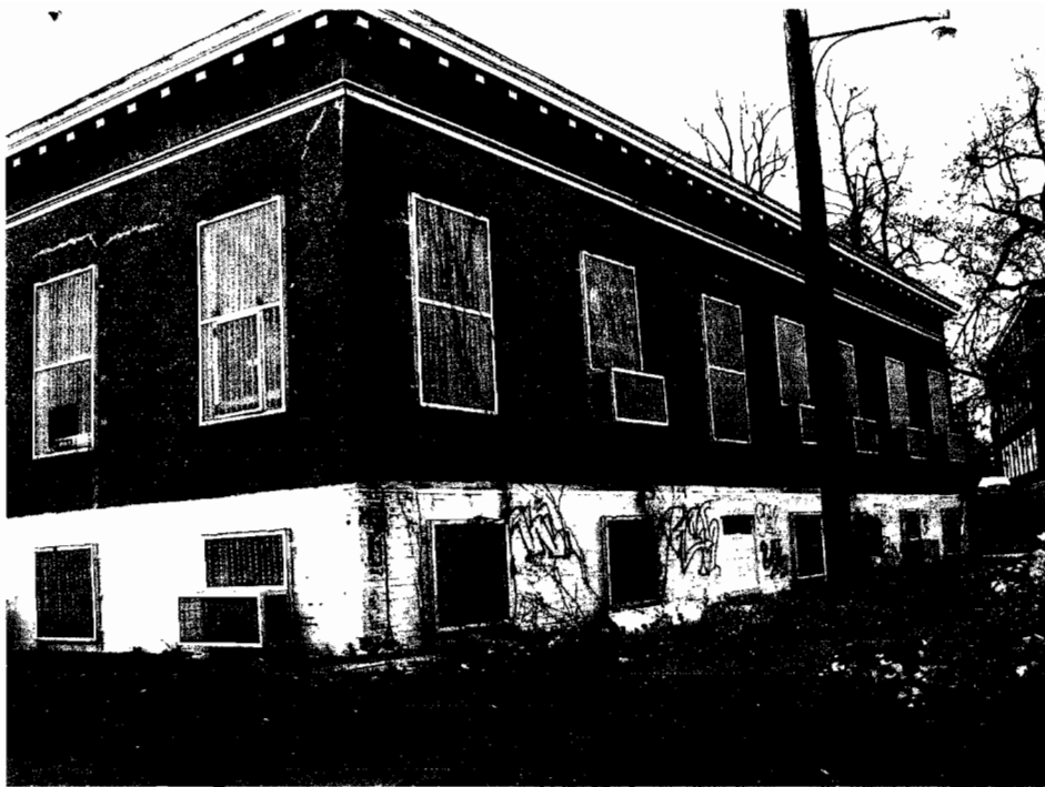
West façade looking southeast
