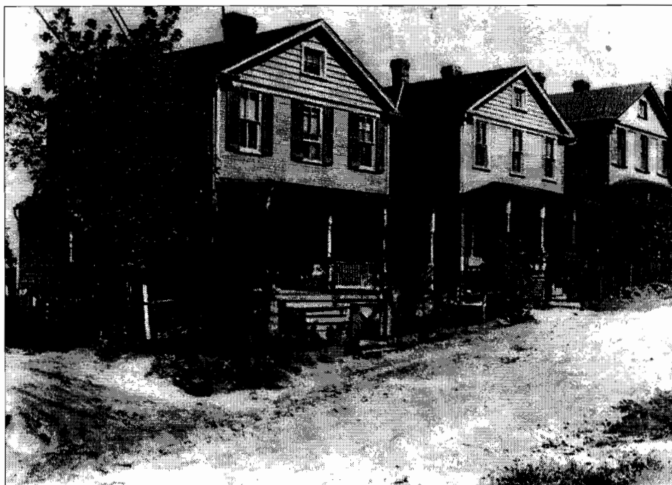
Reno City houses on the north side of Ellicott Street, uphill from Belt Road, photograph from National Park Service, 1930s, reproduced in Helm, Tenleytown D. C. , 201.
