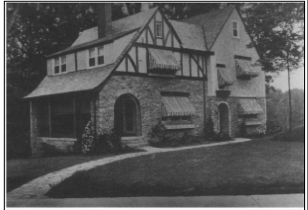
Tudor Revival-style house in Wesley Heights. From "Models of Beauty and Predictability, p. 68.
