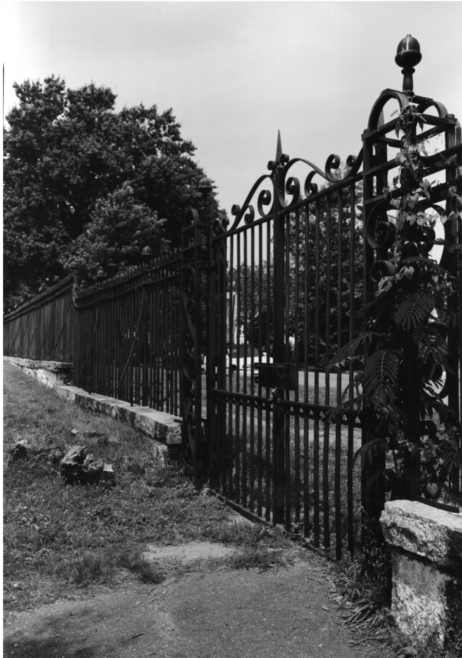
Ceremonial gateway and historic fence along E Street SE on the northern boundary of the cemetery, looking southwest James Rosenthal, HABS, 2005
