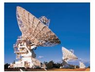
John Mead/Science Photo Library/Photo Researchers Incoming signals are reflected by the parabolic antenna to the receiver at the focus.
