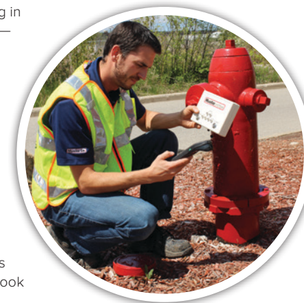
Photo: An Echologics field technician inspects an Echoshore-DX installation situated on a city fire hydrant.
