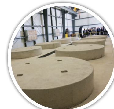
Photo: Ten 250 kW flywheels are stored in a vault at Temporal's Minto, Ontario, installation.
