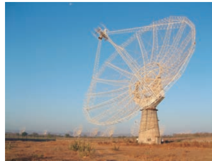
Chapter 3—Fig. 3.8 Fully steerable 45 m paraboloidal dishes of the Giant Metrewave Radio Telescope (GMRT) in Pune, India. The GMRT consists of 30 dishes of 45 m diameter with 14 antennas in the central array. Photograph courtesy: Professor Govind Swarup, GMRT, Pune.
