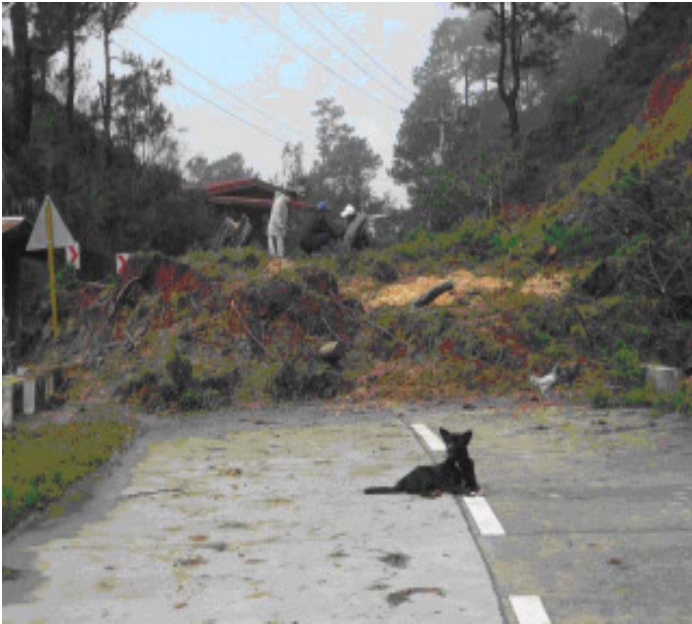
Numerous land slides of this type and other larger ones . Natures wrath while man's best friend sits calmly in the middle of the road. Photo taken on October 10, 2009 along the Ambuclao Road (also known as the Baguio Benguet - Vizcaya Road) . Photo by O. Trazo
