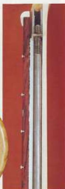
Steel Truss Rod housed in alu- minium channel.
