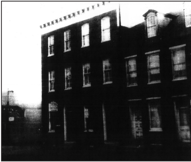
214 West King Street, Lancaster, Pennsylvania, former site of the Water Street Rescue Mission, became home to the Good Shepherd (Hispanic) Mennonite Church.
