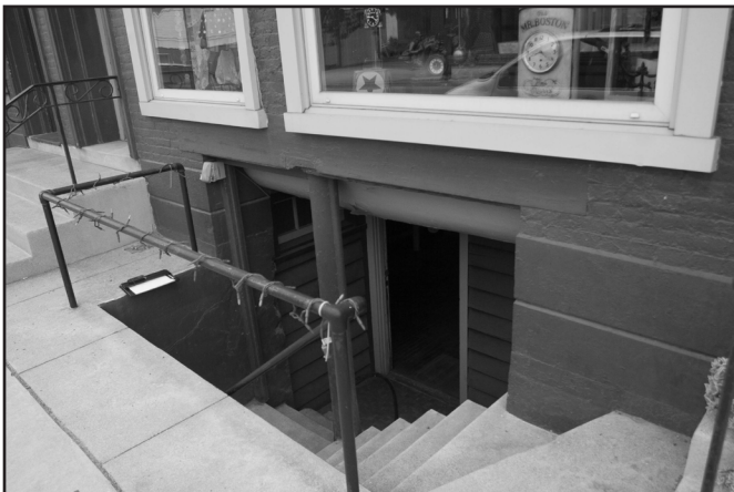
Stairs leading down to one of the first locations of the New Holland Hispanic Mennonite Church, 207 East Main Street, New Holland, Pennsylvania, by Kauffman Hardware
