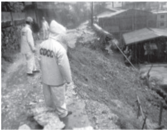
MINA'S PATH OF DESTRUCTION. Volunteers and members of the City Disaster Coordinating Council headed by Action Officer and City Administrator Peter Fianza inspect an eroded portion of road along Upper Pinget barangay asses the damage and put counter measures to prevent further erosion during the height of Typhoon Mina Nov.26.— Photo by Bong Cayabyab
