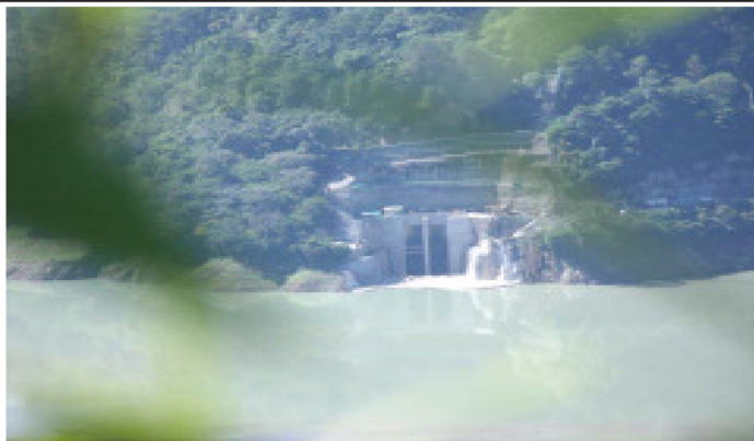
UPGRADED BINGA DAM COMING SOON. The Binga Power Plant in Benguet is currently being upgraded. The refurbishment which began in 2010 will upgrade the plant from 100 megawatts to 120 megawatts one unit at a time within three to four years to supply more power to recipients in the Luzon Area./ Grace Bandy
