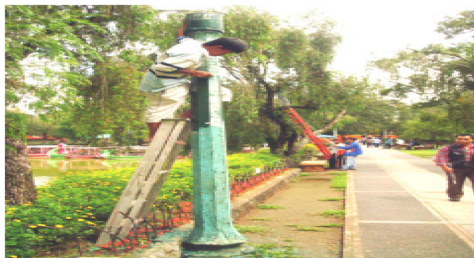
BEATING THE DEADLINE - Department of Public Works and Highways-Baguio District Office laborers work rain or shine to install electrical wirings while the original lamp posts are being restored and rehabilitated for Burnham Park's eco-friendly lighting system.— By Bong Cayabyab
