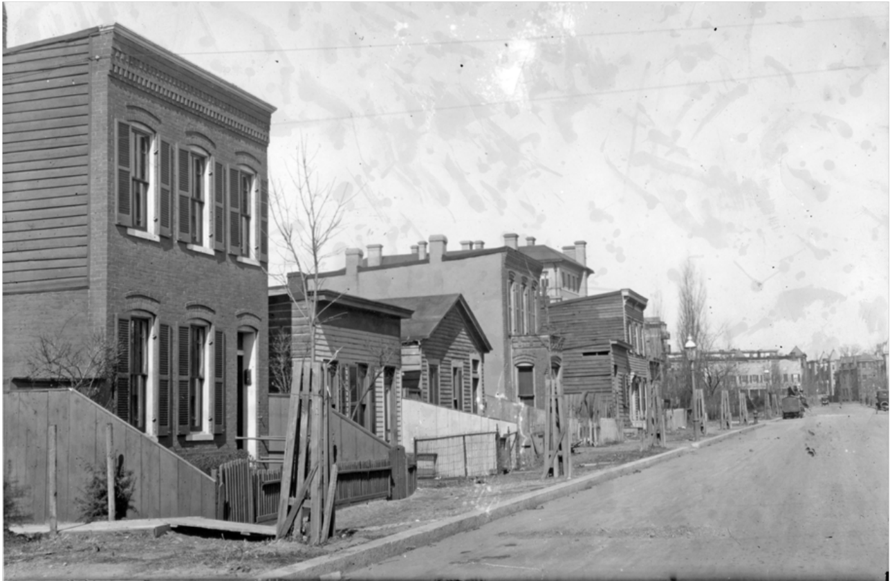
Houses on 15 th Street (Columbia Avenue on plat) in the Meridian Hill Subdivision prior to demolition in 1915. The MacVeagh House (later Embassy of Mexico), built 1910, is visible at the center of photo rising above and behind the still extant frame houses. (Courtesy of Historical Society of Washington CHS 5203)
