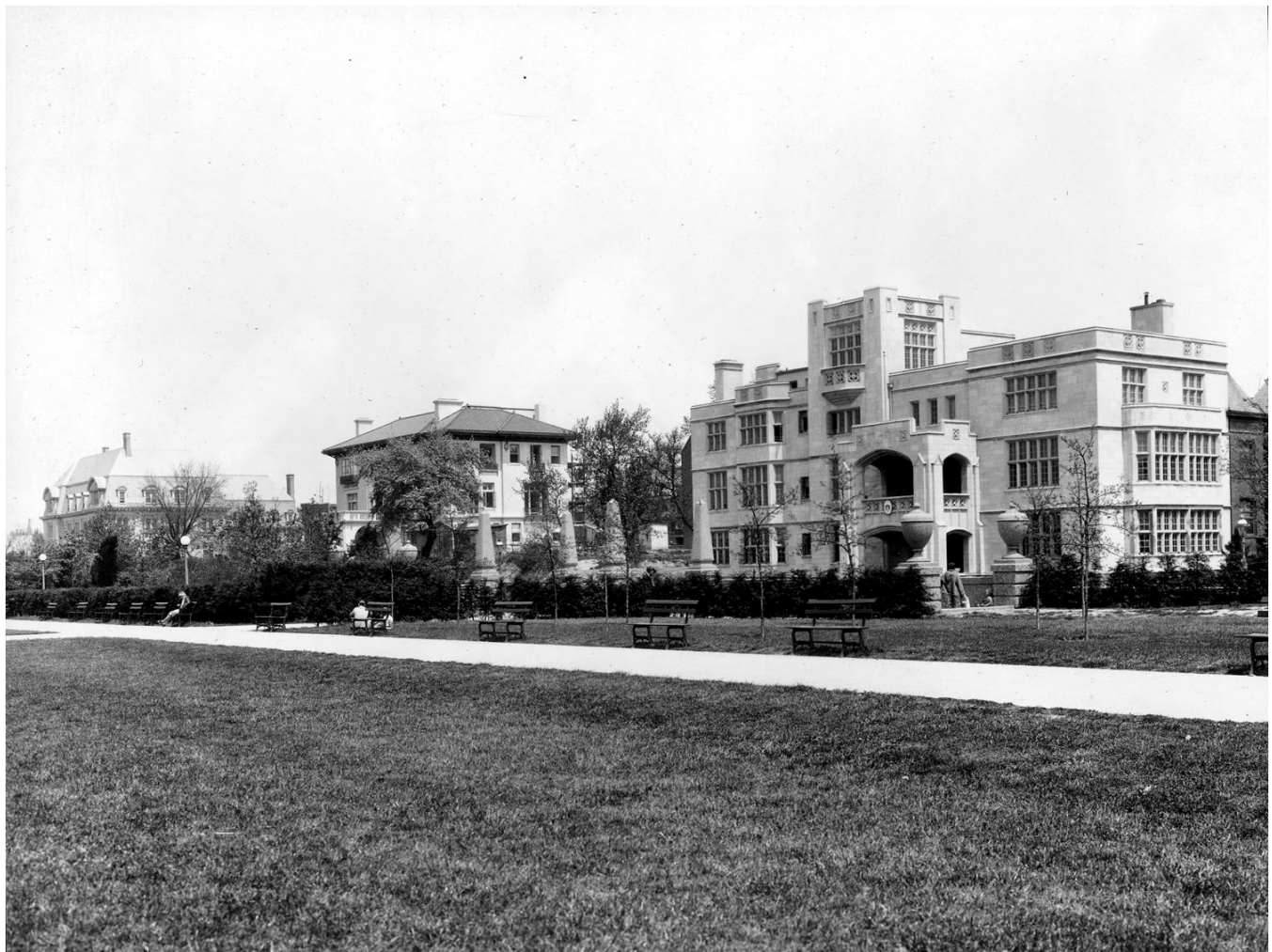
View of 2401, 2437 and 2535 15 th Street looking northeast from upper esplanade of Meridian Hill Park, ca 1925. (Courtesy of the Historical Society of Washington CHS 07677)
