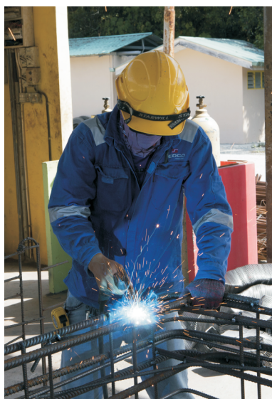
MIG welding for caging
