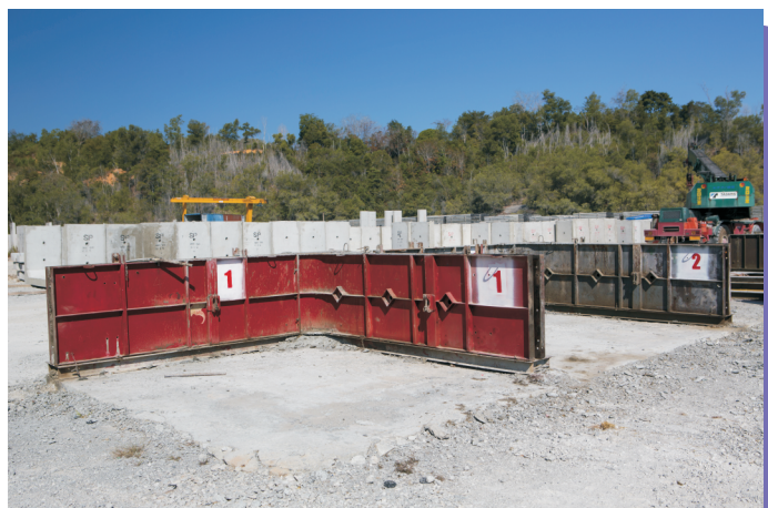
Steel form for dimensional accuracy
