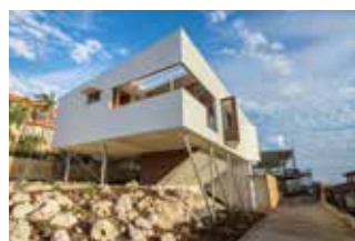
A SUBURBAN BEACH HOUSE 19A Beach Road, Coogee
