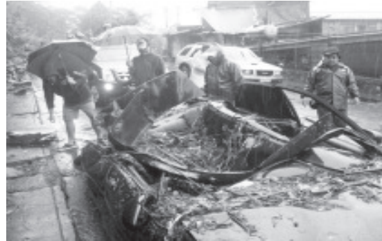
A car was wrecked by an eroded riprap along Ambuklao Road. A van was also slightly damaged on the said area.
