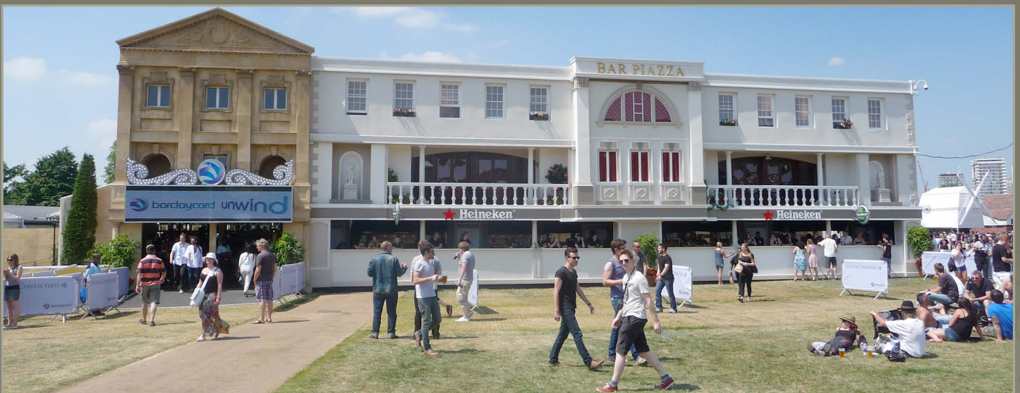
Three storey bar and venue entrance built from nine shipping containers at Hyde Park British Summer Time Festival.
