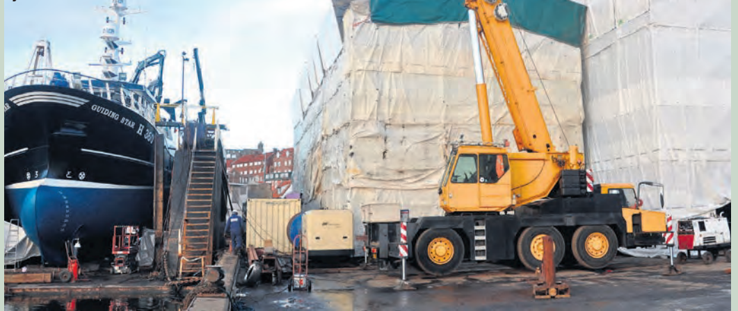
Guiding Star on Parkol floating dock last week while fitting out and machinery installation of another two new boats of similar size continues at the yard
