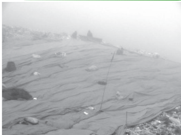
'REMEDIAL MEASURES' – Personnel of the City engineers Office and City Environment and Parks Management Office covers the garbage with tarpaulin to prevent rain water from seeping in during the height of Typhoon Pedring at the Irisan Controlled Dump Facility./Photo by prillorta
