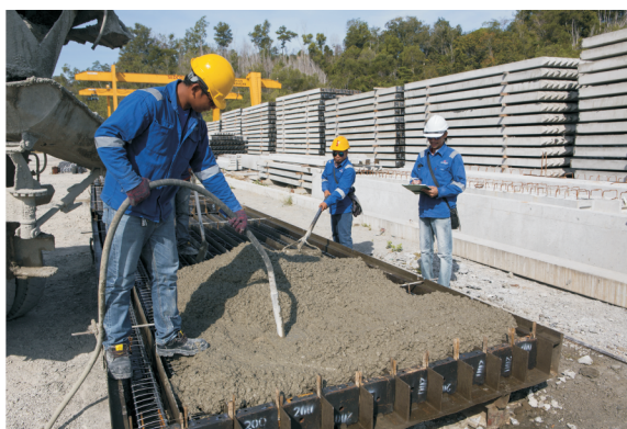
Production In Progress
