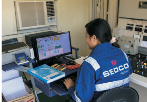
Computerised Batching Plant
