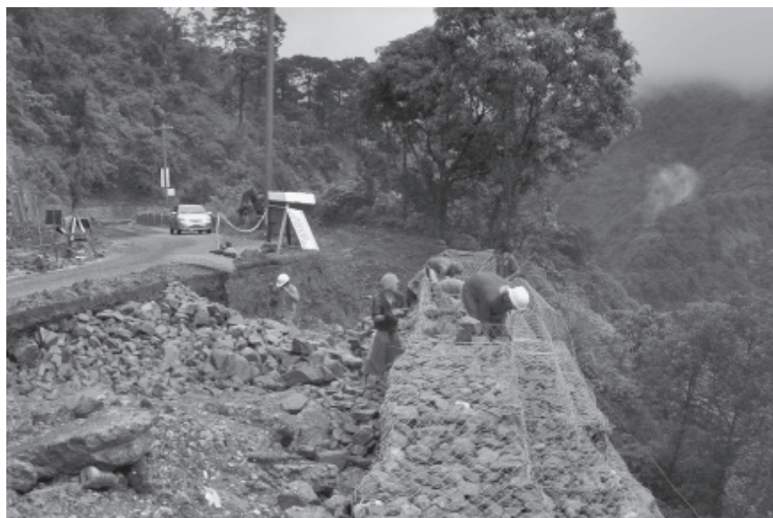
Laborers work despite the inclement weather to finish the retaining wall along the Uabac Section of Kennon Road. /RMC-PIA CAR
