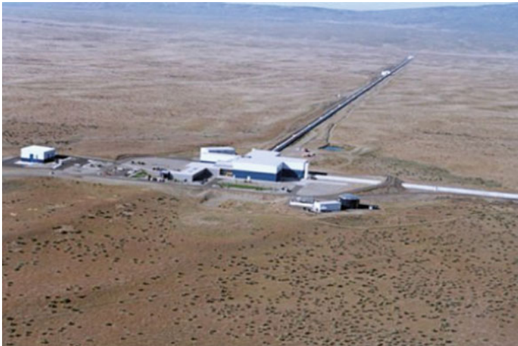
Fig. 18.16 The LIGO interferometer being built to detect gravitational waves. Squeezed light is expected to be used in the interferometer for increasing the sensitivity of the sensor. (Source: Ref. http://physicsworld.com/cws/article/news/33755 )
