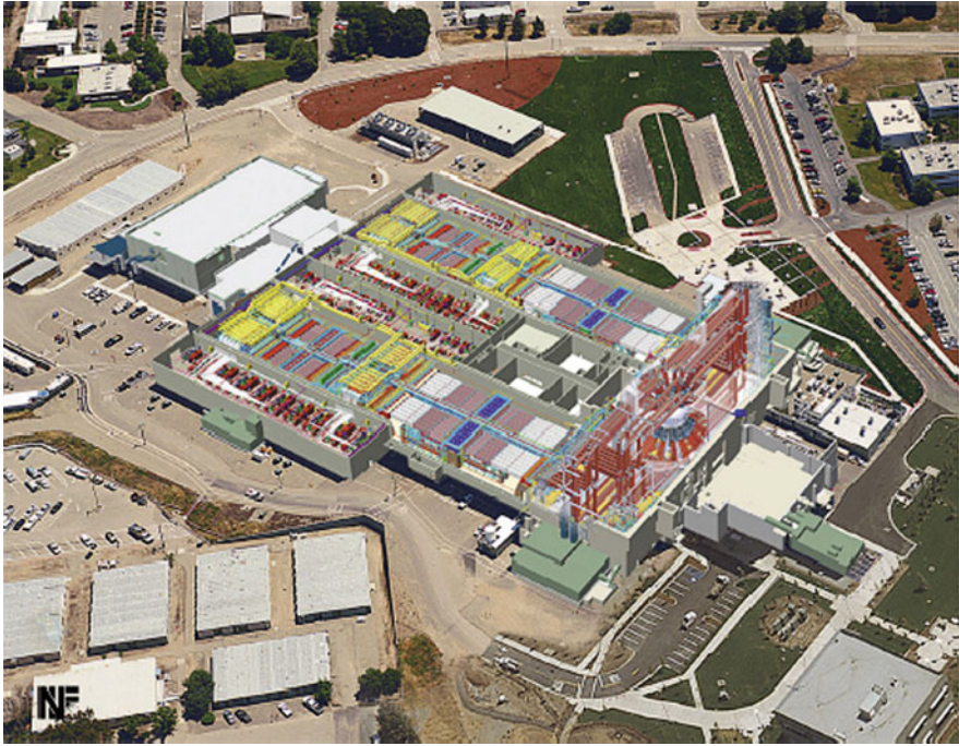
Fig. 16.5 A bird's-eye view of the NIF facility shows the main 705,000 ft 2 building. The structure includes two laser bays capable of generating more than 4 MJ of infrared laser light; four capacitor bays (which store about 400 MJ of electrical energy); two switchyards, which direct all 192 laser beams into the target bay; the target bay, where experimental activities are conducted; the target diagnostic building, for assembling and maintaining diagnostic equipment for experiments; and the Optical Assembly Building ( upper left ), where optics assemblies are prepared for installation. (Source: Rick Sawicki Interview for Dartmouth Engineer Magazine, May 27, 2008)
