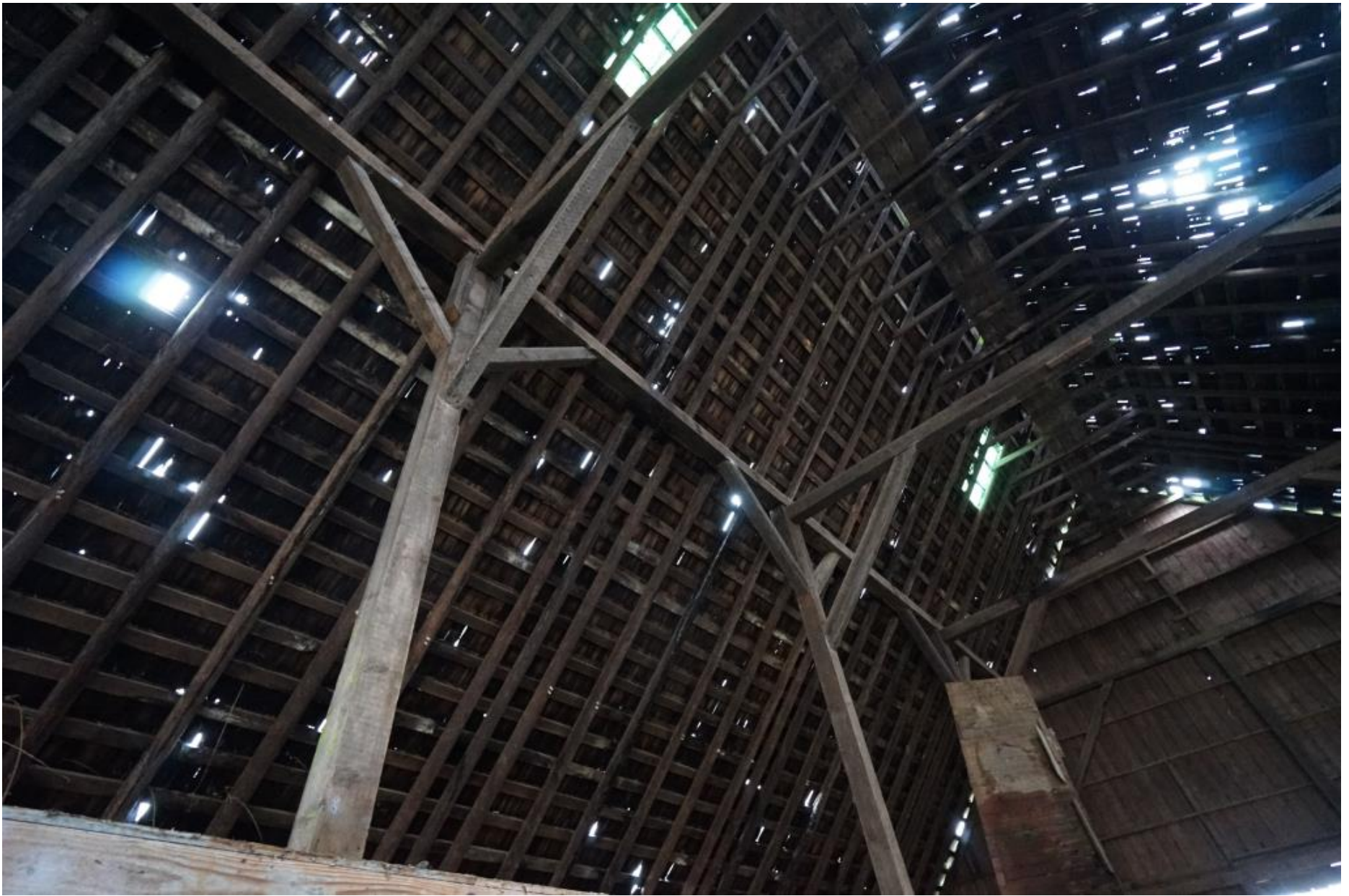
Image of post-beam connections.
