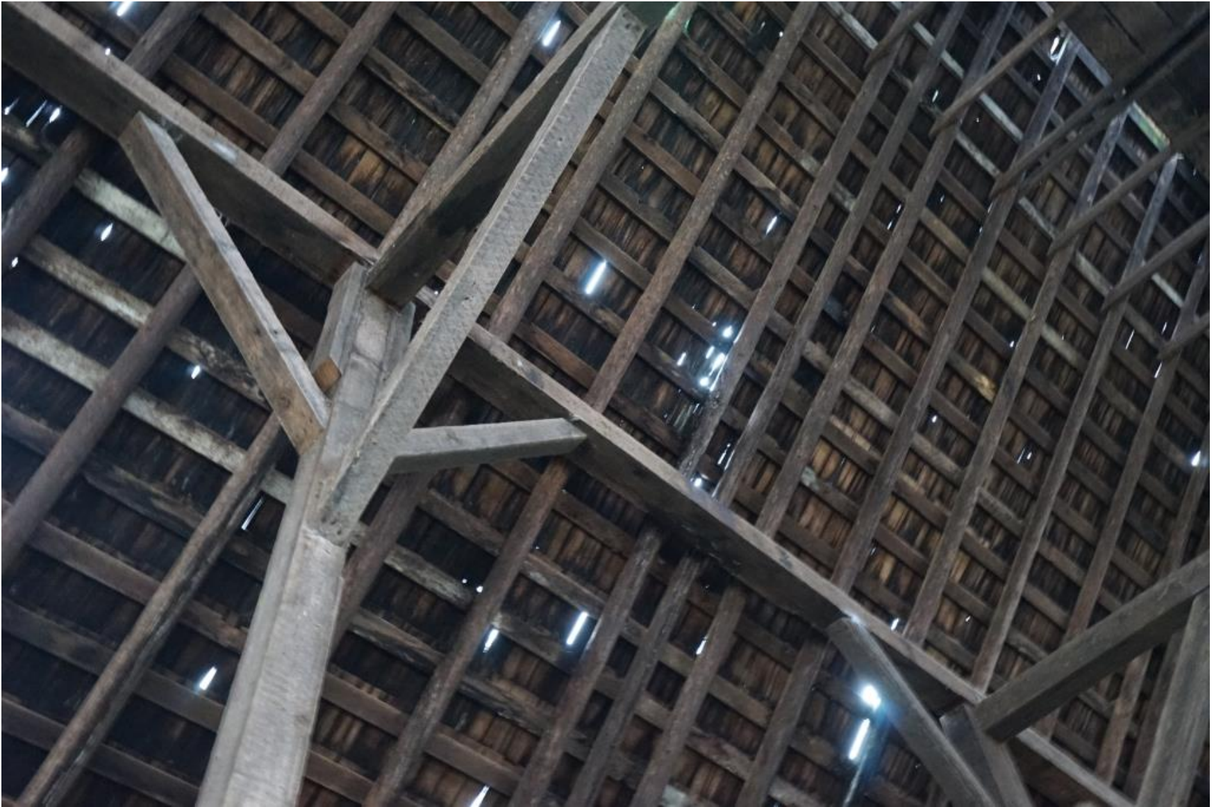
Detail of post-beam connection, showing round-log purlins in roof structure.
