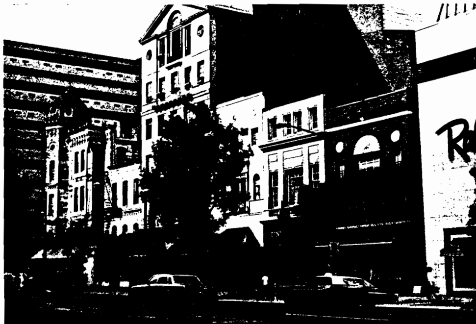
Demonet building, Connecticut Avenue and M Street, N. W., from northwest, August, 1977
