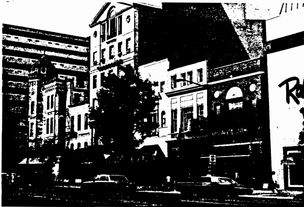
Demonet building, Connecticut Avenue and M Street, N. W., from northwest, August, 1977
