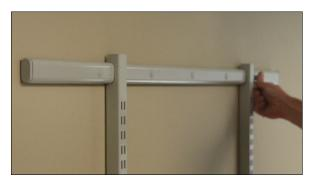
**STEP FOUR:** Insert end caps and hole plugs for a clean finish.
