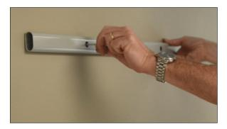
**STEP TWO:** Attach horizontal rail to wall with provided bolts. Be sure to mount horizontal rail with smaller bolt holes touching the wall and large holes facing out. The oval horizontal support rail has mounting holes spaced 8" on center to allow the rail to be attached to the wall structure of the building. It is recommended that the rail be attached to the wall structure in at least two places per every 48".
