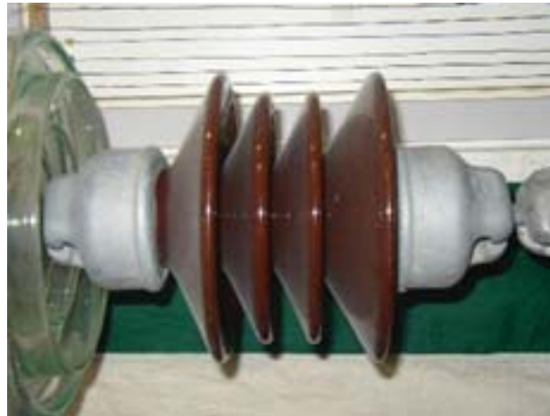
Suspension insulator
