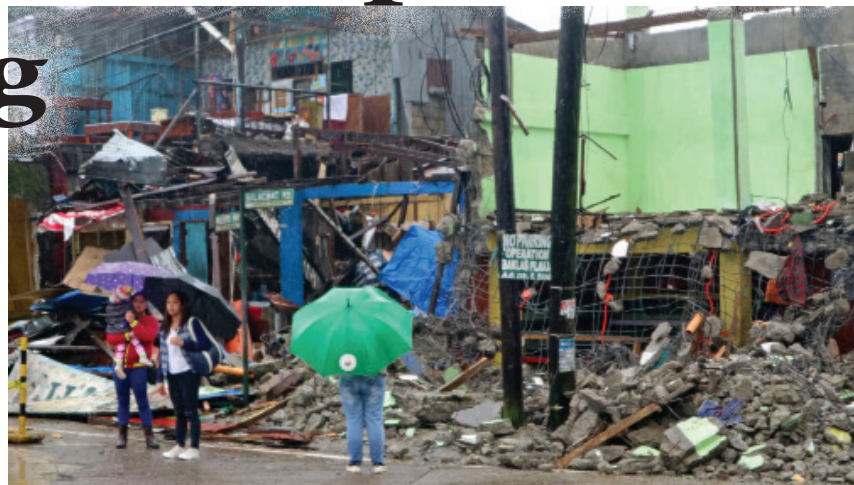
DEMOLISHED - Illegal business building establishments along Marcos Highway were torn down by the demolition teams from the Department of Works and Public Highways, City Engineers Office and the City Buildings and Architecture in compliance to the national direction to clear road-right-of-ways from encroachments and obstructions. - By Bong Cayabyab
