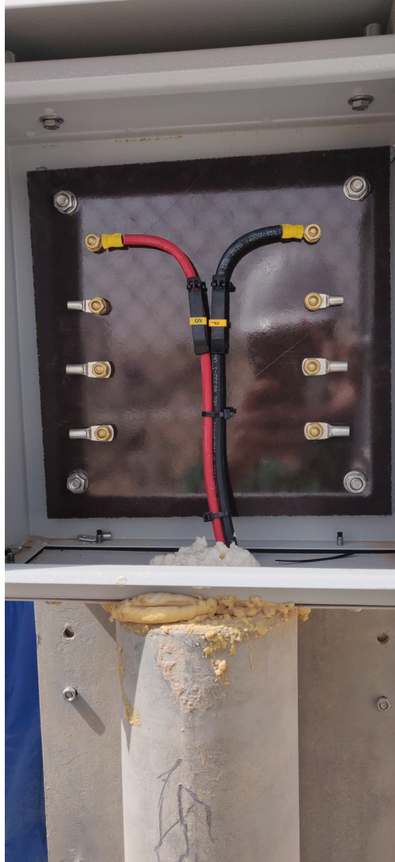
Figure 26: Measuring the \Delta V between in station DSS and out-of-station CS.
