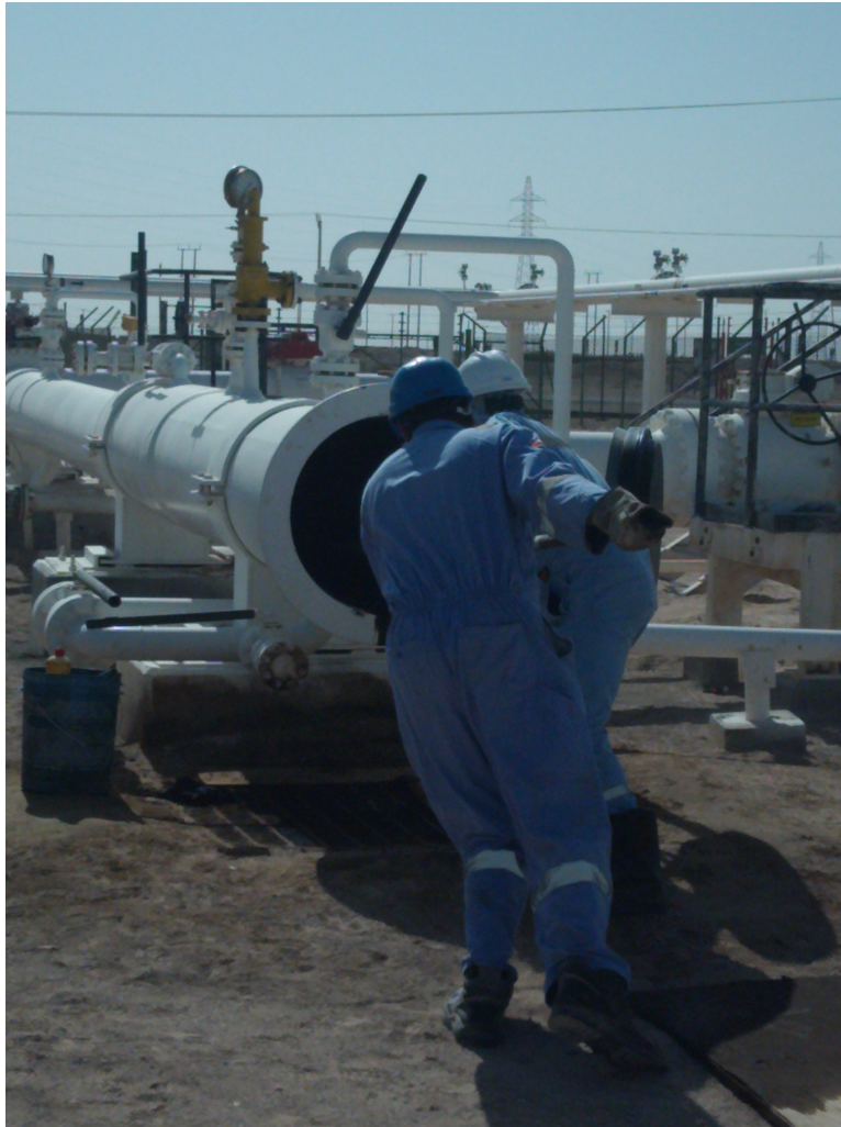
Figure 16: Pushing the pig into the launcher
