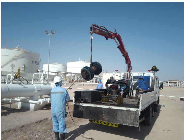
Figure 15: Loading the pig into the launcher
