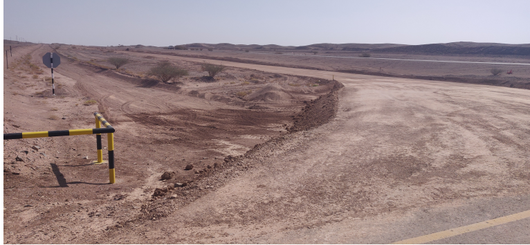
Figure 27: R.O.W unauthorized disturbance
